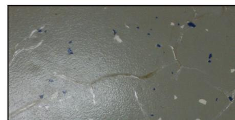
In some applications, problems may arise resulting in wrinkling of the coating that was previously applied to the floor.
