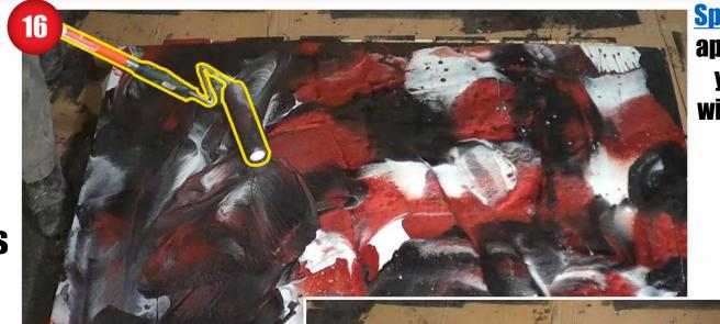
Spike shoes are ESSENTIAL when applying floor epoxy. They allow you to walk on the wet epoxy without ruining the pattern, and help with slip resistance
