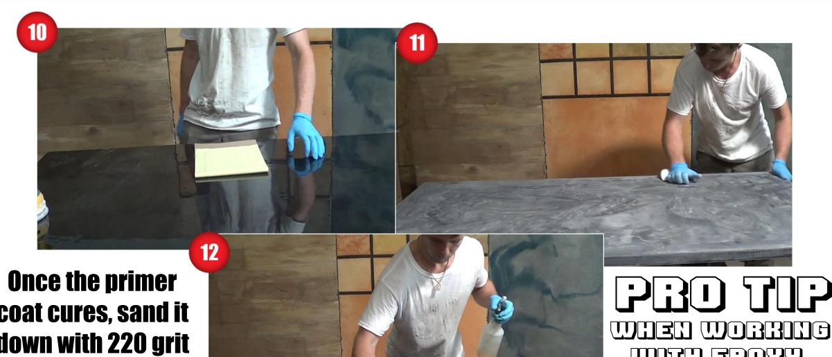
once the primer coat cures, sand it down with 220 grit sanding paper, and wipe it down with denatured alcohol
