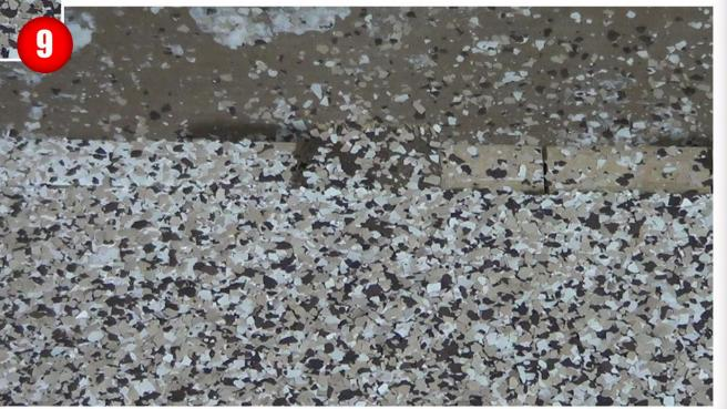
Once the <u>epoxy</u> dries, (usually 12-24 hours) vacuum the extra <u>flakes</u> off
