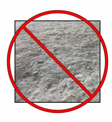
**Make sure your** floor is completely flat and level. This can be achieved with a floor grinder or self leveling concrete.
