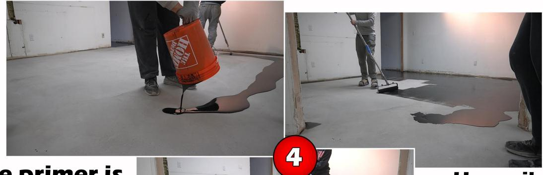
The primer is spilled and rolled out on your vacuumed floor
