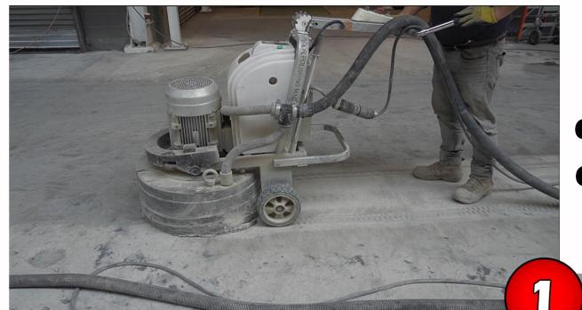
The floor must be grinded to remove the top layer of concrete so that the epoxy can properly adhere to the floor
