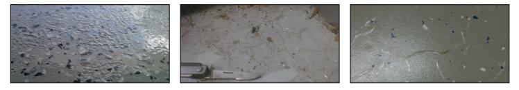
In some applications, problems may arise resulting in wrinkling of the coating that was previously applied to the floor.
